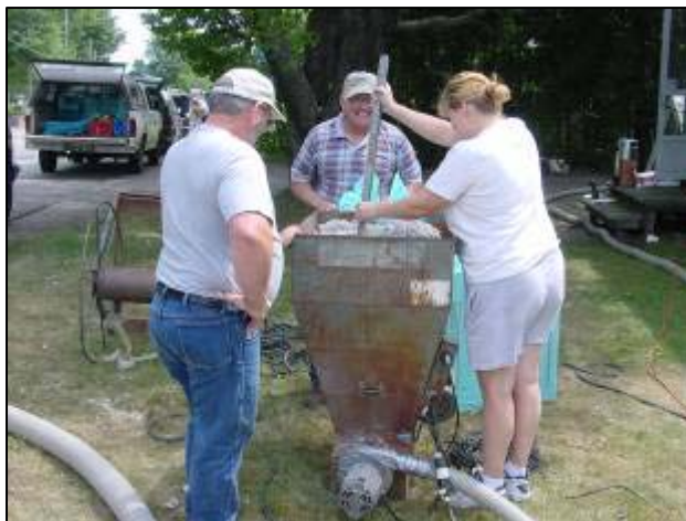
Readying cellulose for wall blow in Maine
