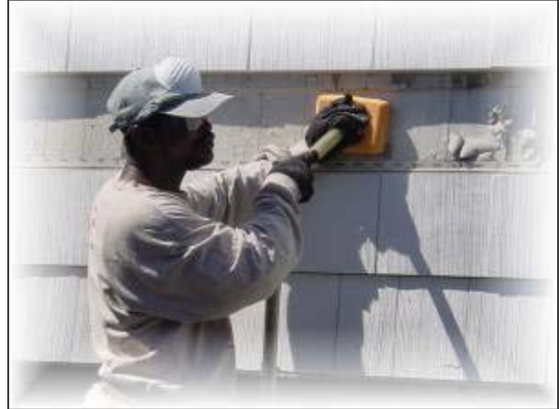
Dense blowing in Connecticut
