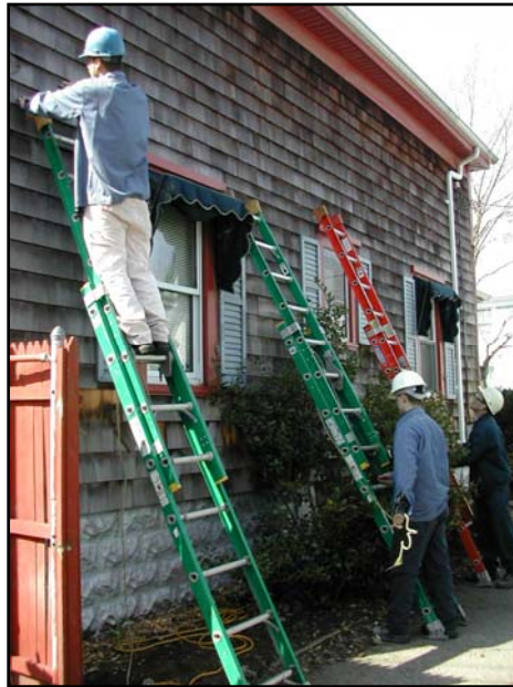
Preparing a wall in Massachusetts, O 4 S Pilot Project
