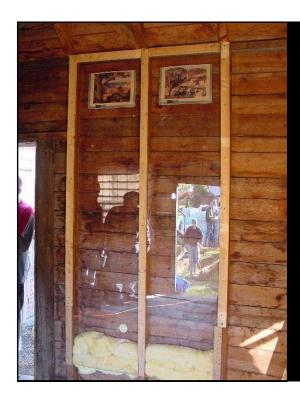
Two 22 inch wide cavities, ¼ inch Lexan, strapped for strength. Fiberglass stuffed in bottom of cavity. Cavities are 3 ¾ inches deep.
